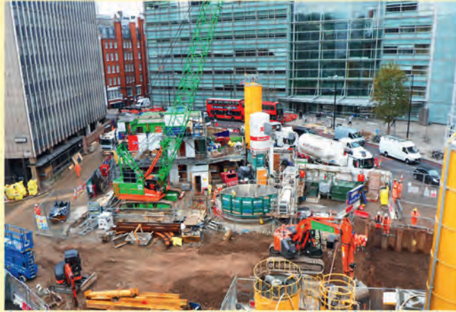
A rail construction site in London analysed by NoiseMap
