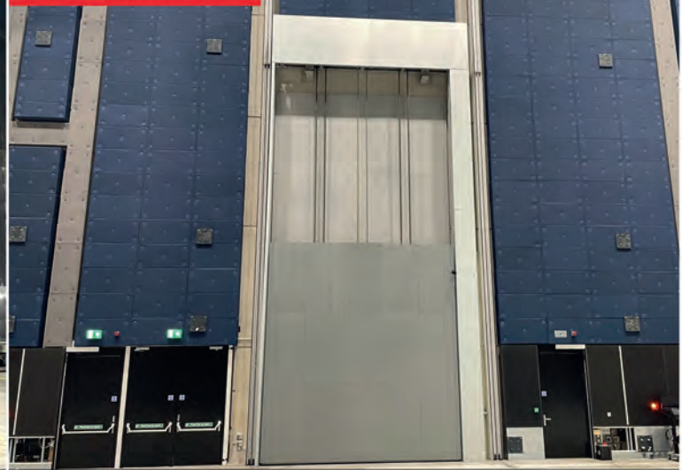
Vertical composite leaf sliding acoustic access door from Rw41dB to Rw58dB
