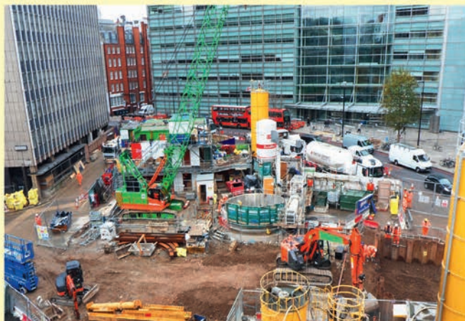
A rail construction site in London analysed by NoiseMap
