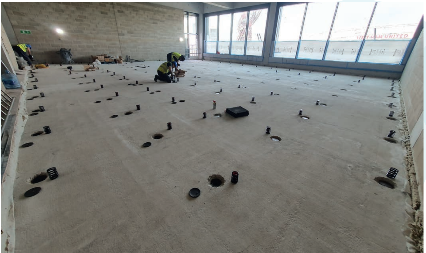
Above: Inserting the floating floor springs before commencing jacking, to within 5mm across the whole area
