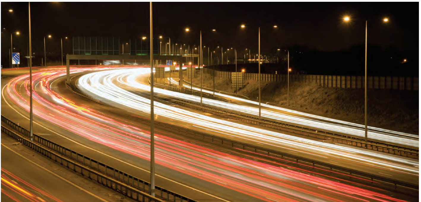
It is important to check that the test arrangement for acoustic performance of the barrier being assessed matches the actual in-situ conditions
